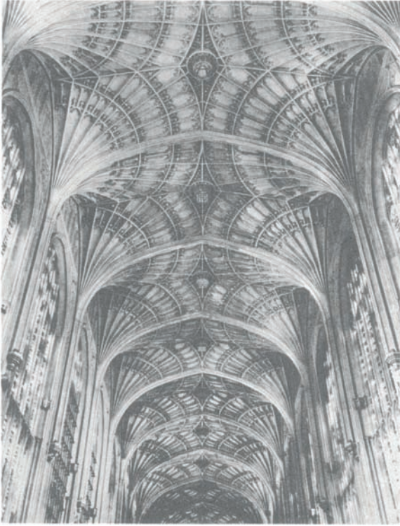
FIGURE 2. The ceiling of King's College Chapel.
